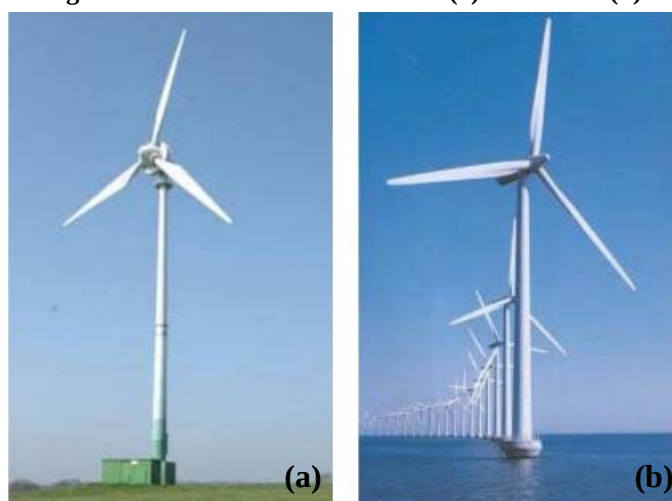
Figura 9 – Turbinas eólicas on-shore (a) e off-shore (b).
