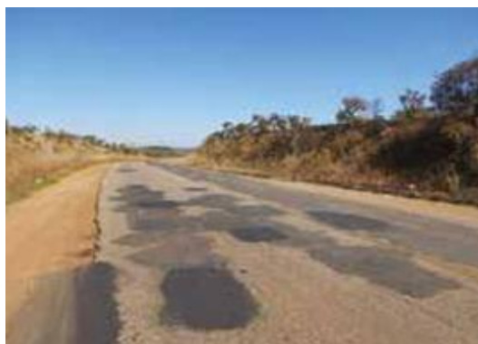
Figura 11 – Remendo
