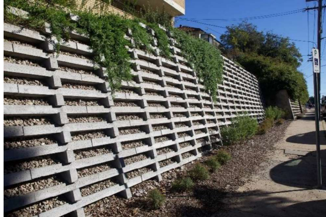
Figura 4 - Muro Crib Walls
