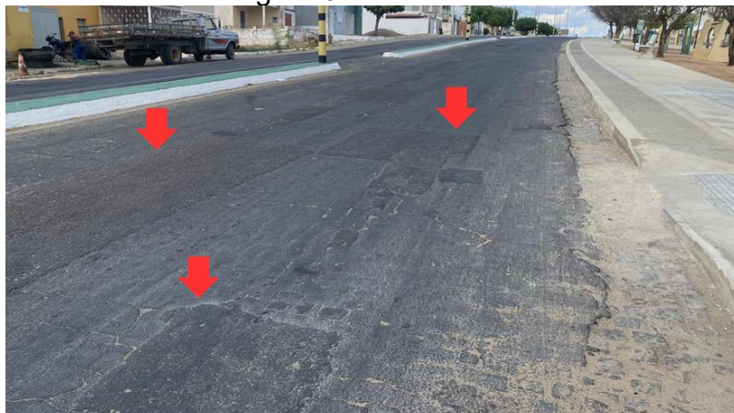
Figura 31 – Remendo
