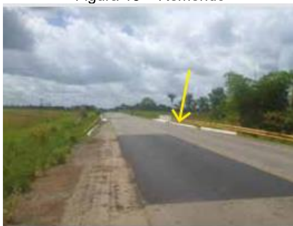
Figura 15 – Remendo
