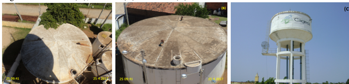
Figura 7 – RAP-01(A), RAP-02(B) e REL-01(C).
