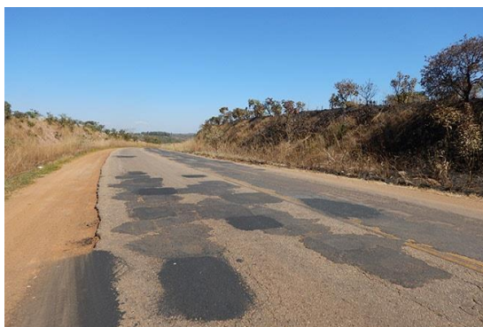
Figura 15 – Remendos
