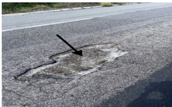
Figura 6 – Panelas (P)
