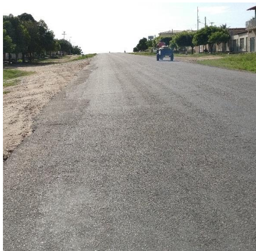
(a) Trecho 1 – RN 233
