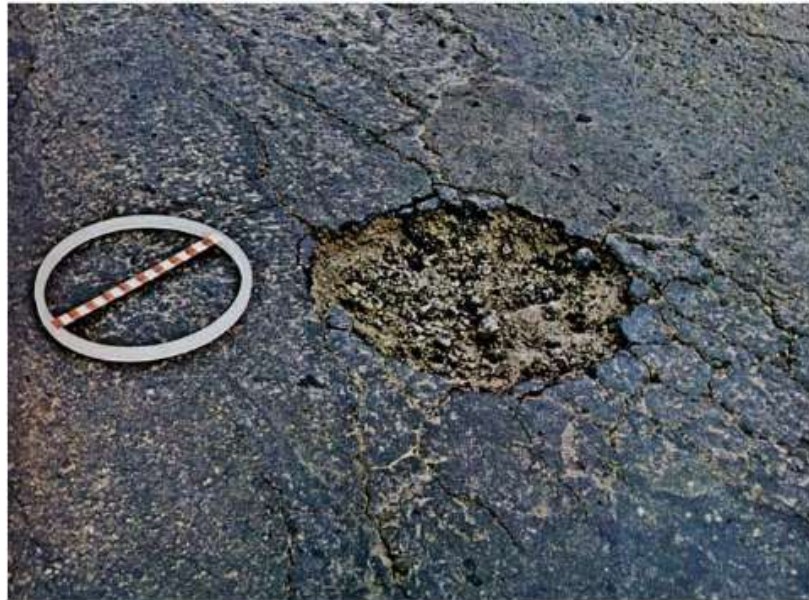
Figura 14 – Panela/Buraco
