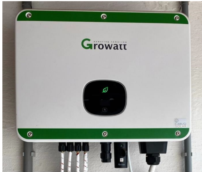
Figura 6 - Inversor solar Growatt on grid MID15KTL3-X
